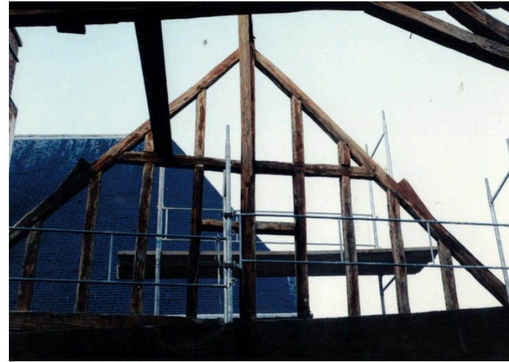
Pendant travaux During construction
