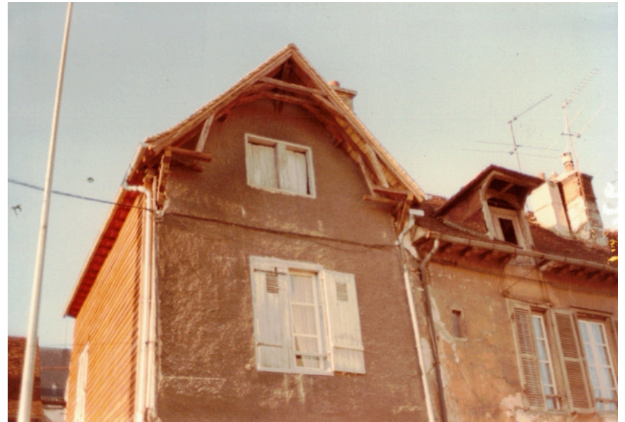
En cour de restauration (1982) Undergoing restoration (1982)
